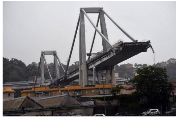
Fig. 7. Central part of crashed Viaduct Morandy
