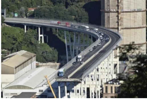
Fig. 6. Viaduct Morandy in Genova-Italy after the crash - Genova
